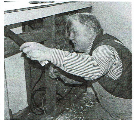
Gary Burch tears out drywall around Community Room windows
